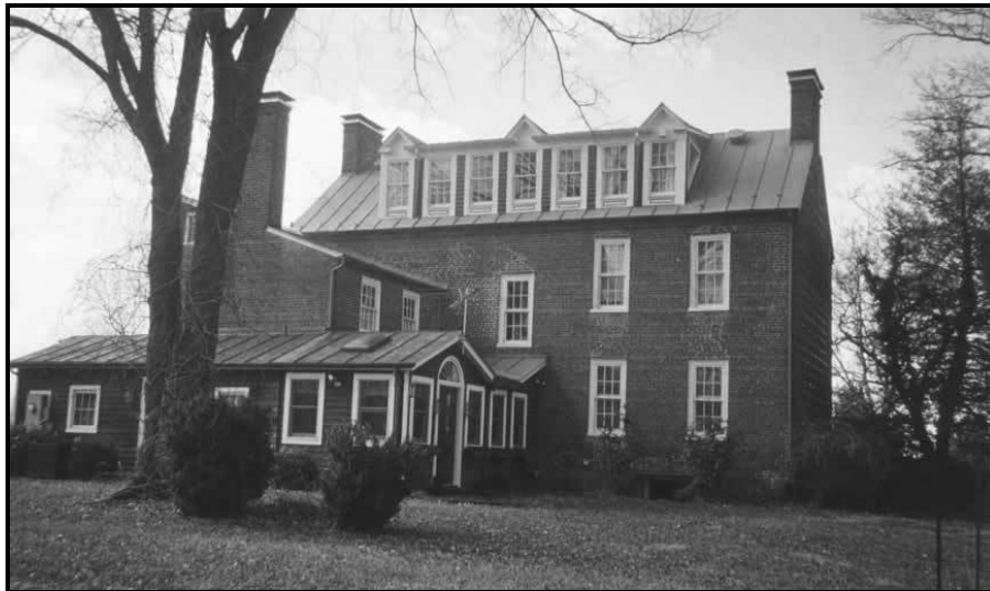
Back View of Moor Green
